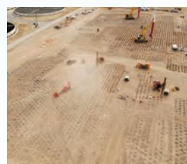
Wick drains have been installed and are being monitored on the site where additional soil has been placed. These geotextile filter-wrapped plastic strips with molded channels provide
