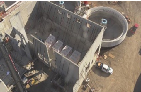
Blower Building and Gravity Thickeners
